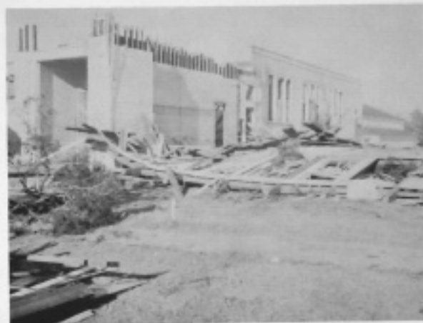
THE OLD HIGH SCHOOL BUILDING
