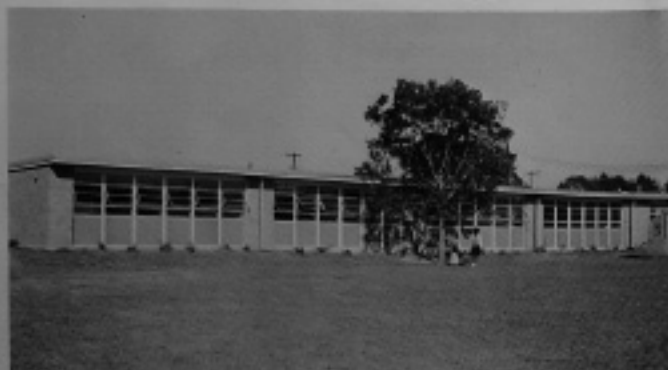
The new wing
