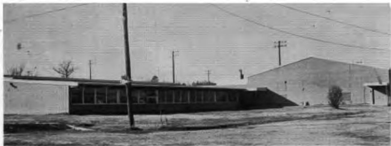
Side View — Classrooms and Gym.
